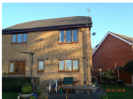
4. Rear of application property
